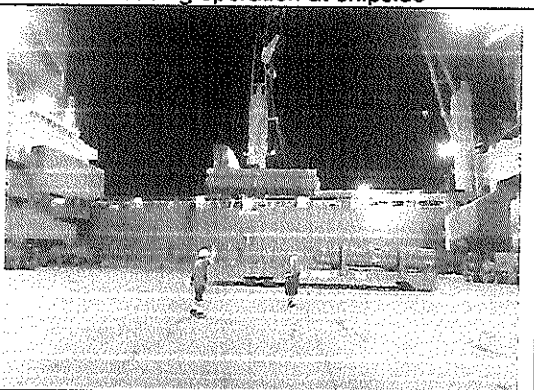
Loading operation at shipside
